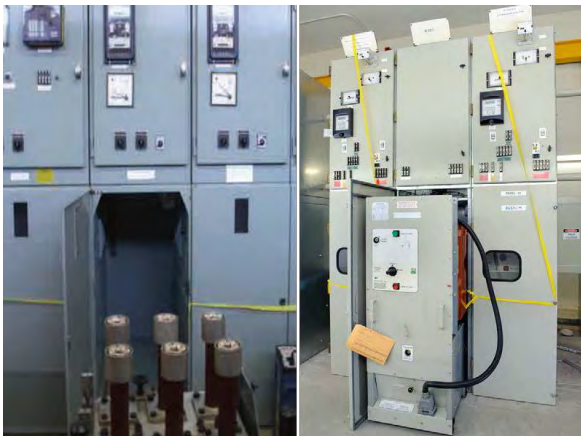
Examples of multi-panel taping Indoor Switchgear for Barrier-out Method.
