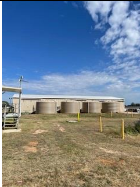
Photo 12: Rainwater storage tanks and fire connection
