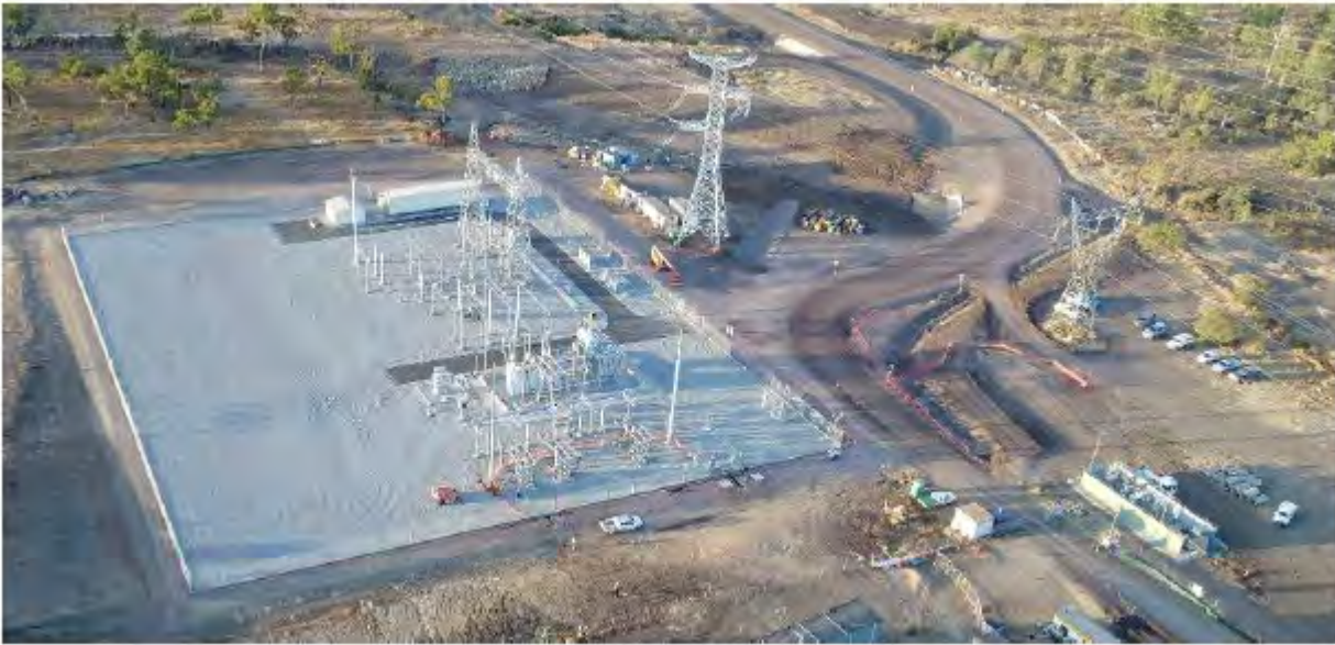
Figure 2-11 Substation under construction (example) (Source: Edify Energy, 2020)
