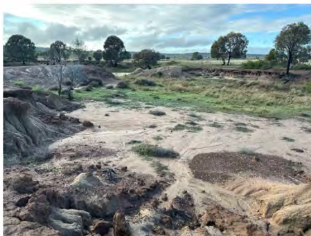
Across vegetation with adjacent dam
