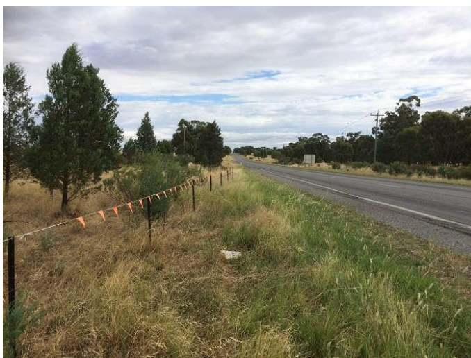
Figure 14 Example of exclusion zone fencing/flagging
