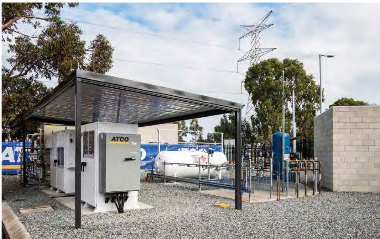
Compressed hydrogen storage tank and gas blending pipes at ATCO's Clean Energy Innovation Hub in Jandakot. Image attribution: ATCO.
