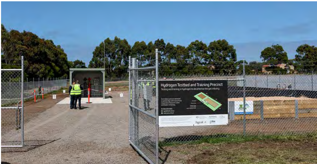
Hydrogen testbed and training precinct. Image attribution: Deakin University.
