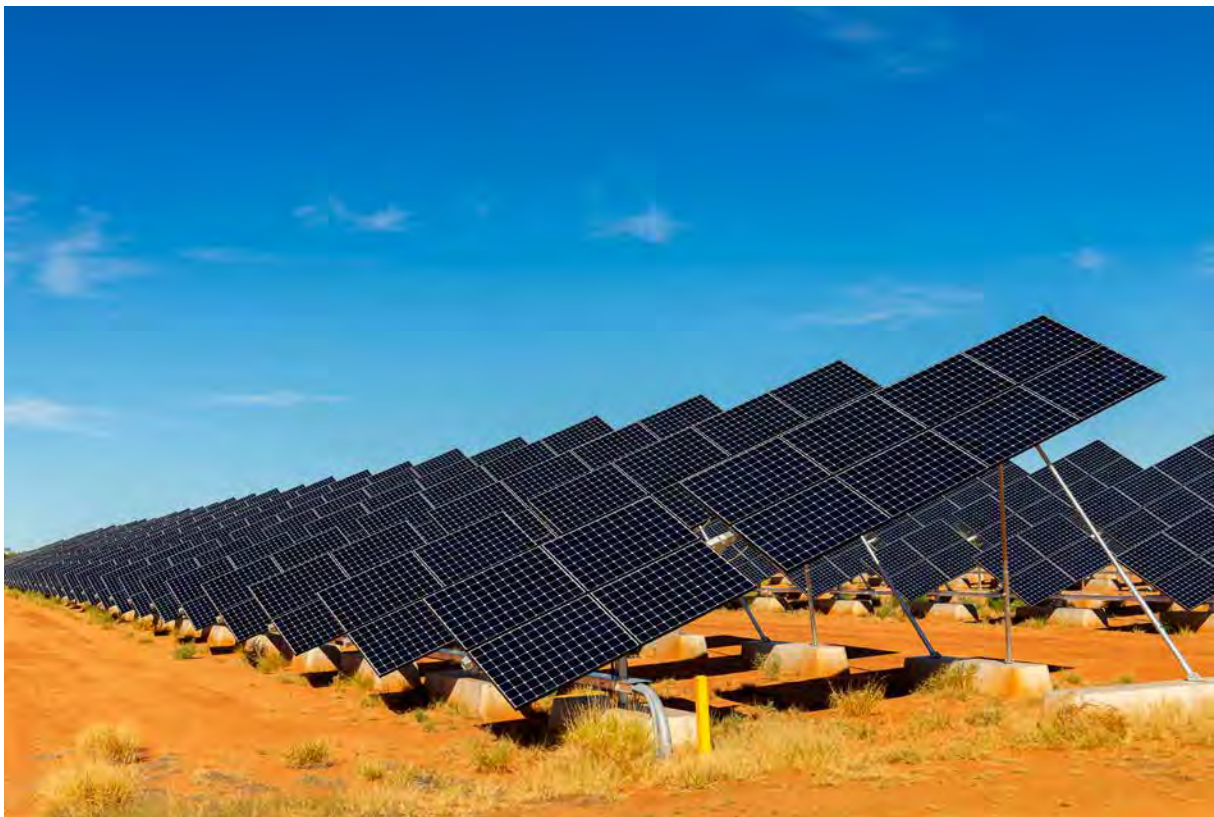
Uterne solar power station near Alice Springs. Image attribution: Gettyimages Christopher Groenhout
