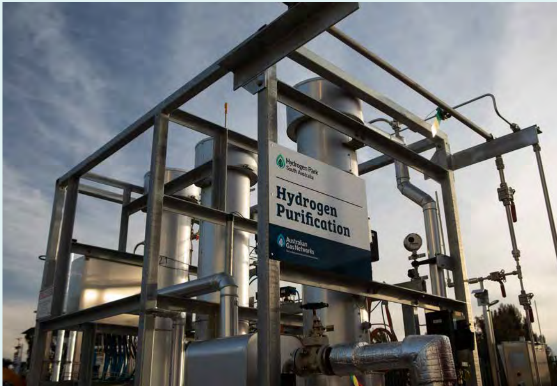
Australian Gas Networks – Hydrogen Park South Australia (HyP SA). Image attribution: Australian Gas Infrastructure Group.
