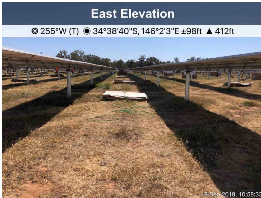
Photograph 62: Waste piles collated at point of install ('Golden Row'), to reduce movement of wastes
