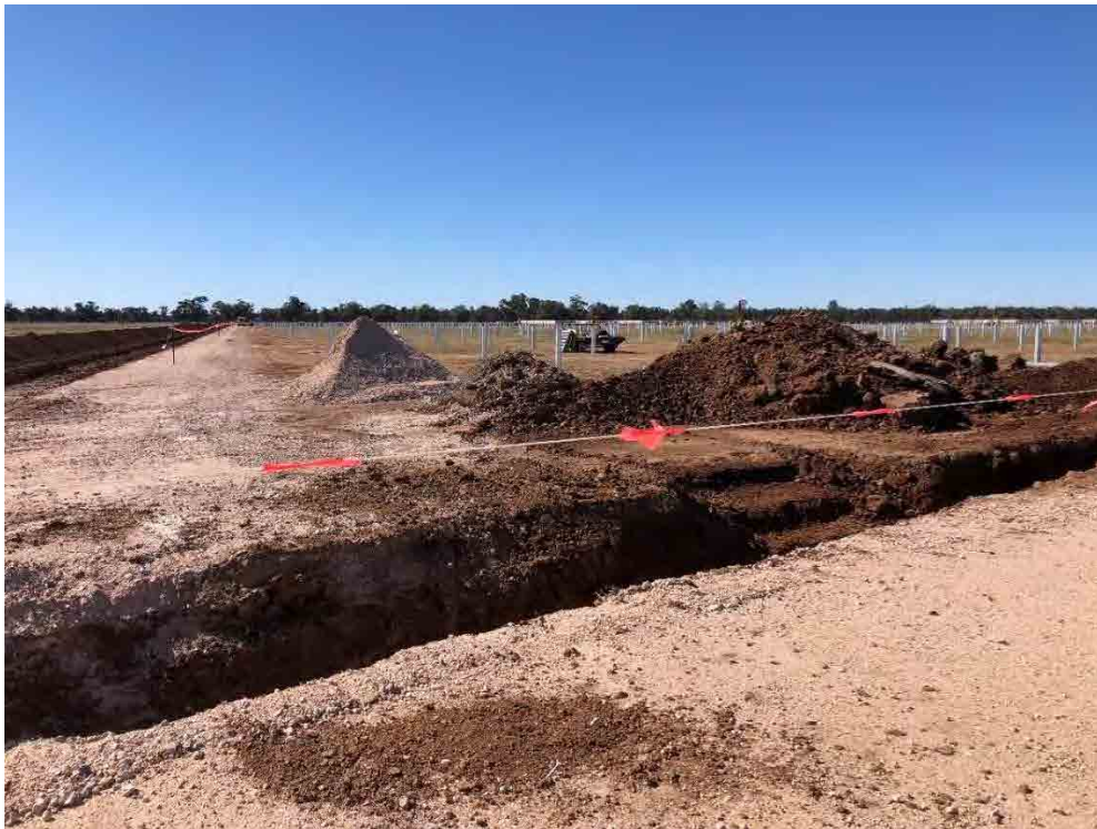
Photograph 2: Open cable trenches and uncontrolled stockpiles, benched ramp for access/egress
