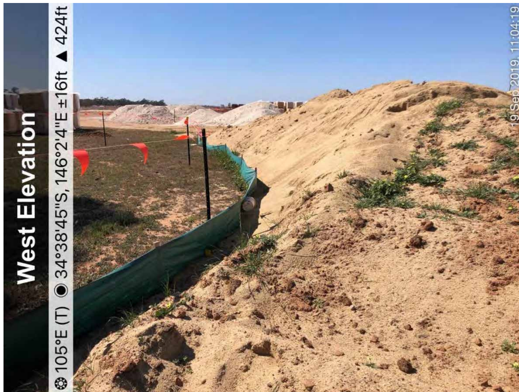
Photograph 66: ESC around large sand stockpile near front entrance satisfactory, may need to cover if not utilised in near future
