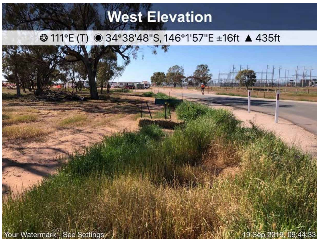
Photograph 49: Northern drain at front entrance, ESC devices and vegetation to filter runoff
