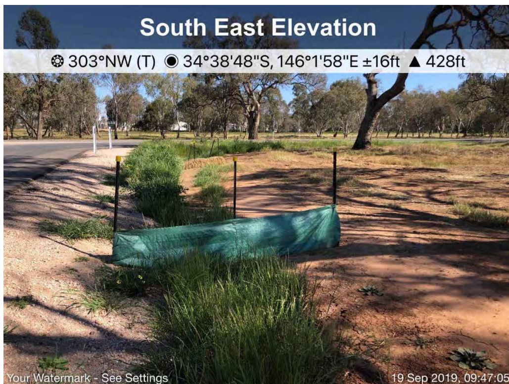
Photograph 51: Northern drain at front entrance, view to front, ESC device recommended to remove or replace with rock filter, coir log or hay bale, adequate vegetation to filter runoff
