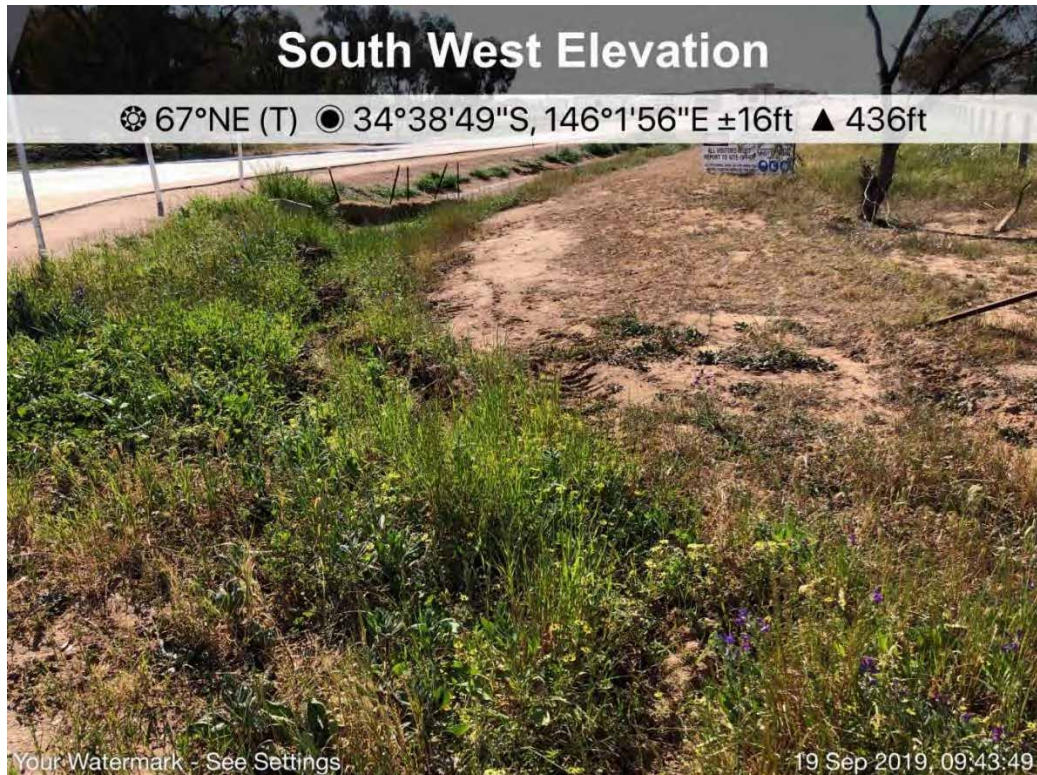
Photograph 47: Southern drain at front entrance, ESC device and vegetation to filter runoff
