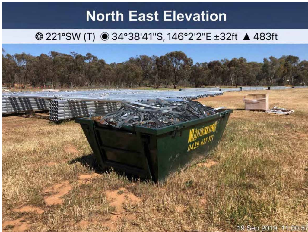
Photograph 64: Metal waste skip, located near to point of 'Golden Row' installation to reduce movement of wastes and increase compliance with waste separation
