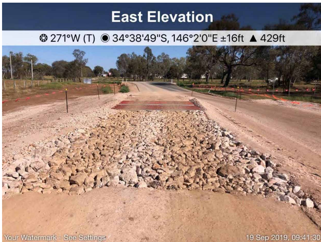
Photograph 43: Rumble pad and grid at front site entrance
