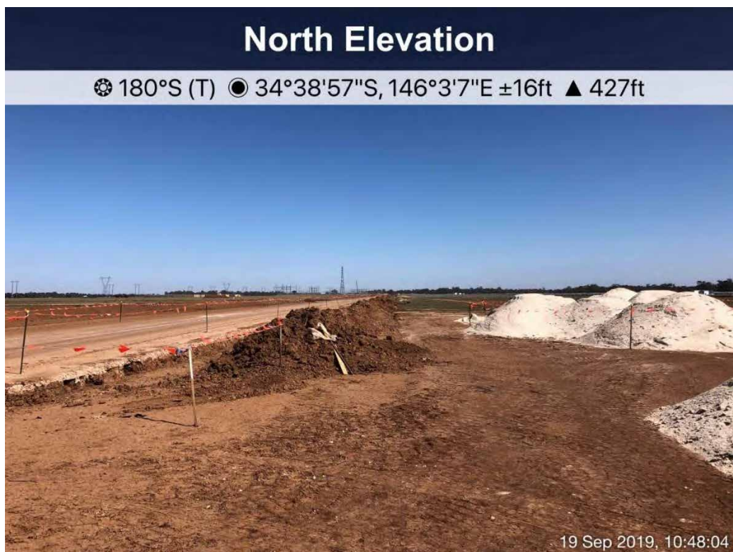
Photograph 59: Sand and topsoil stockpiles, not adequately protected with ESC devices
