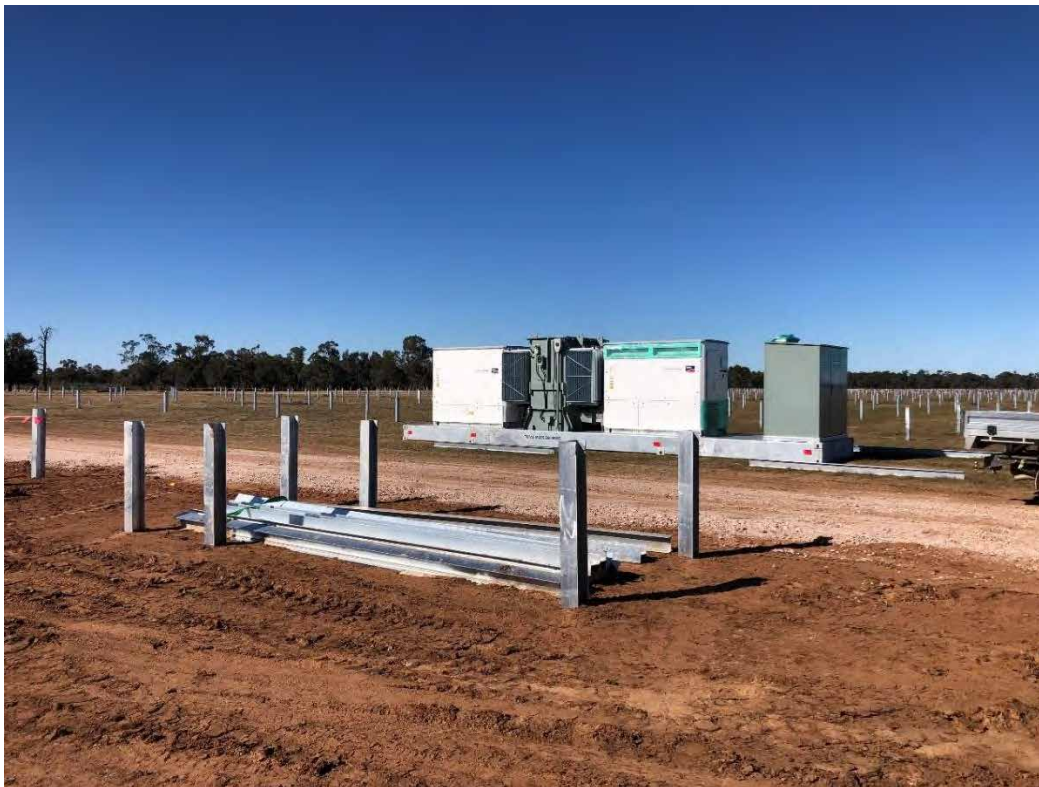
Photograph 4: PCU area prepared for lifting/mounting PCU, Note: pile installation in background
