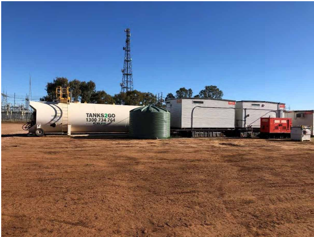
Photograph 16: Diesel self-bunded storage tank, located at edge of compound
