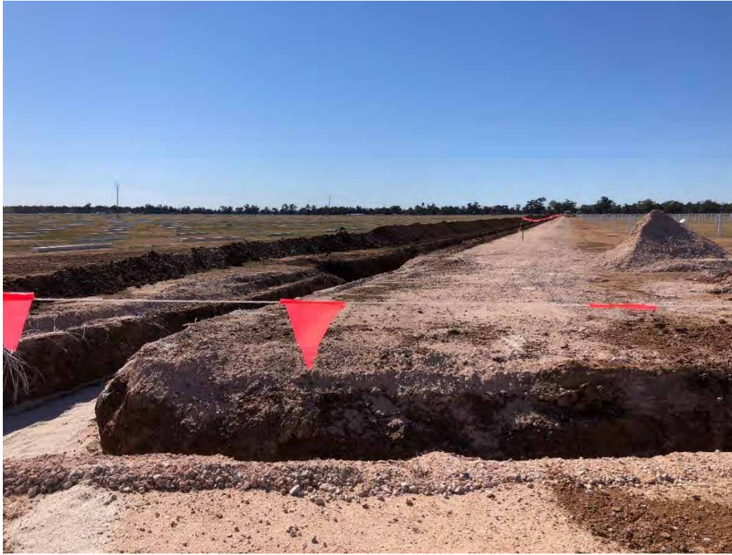
Photograph 3: Typical view of open cable trenches throughout the site, benched access/egress ramps visible
