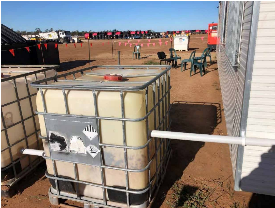
Photograph 22: IBCs plumbed to toilets to collect septic waste
