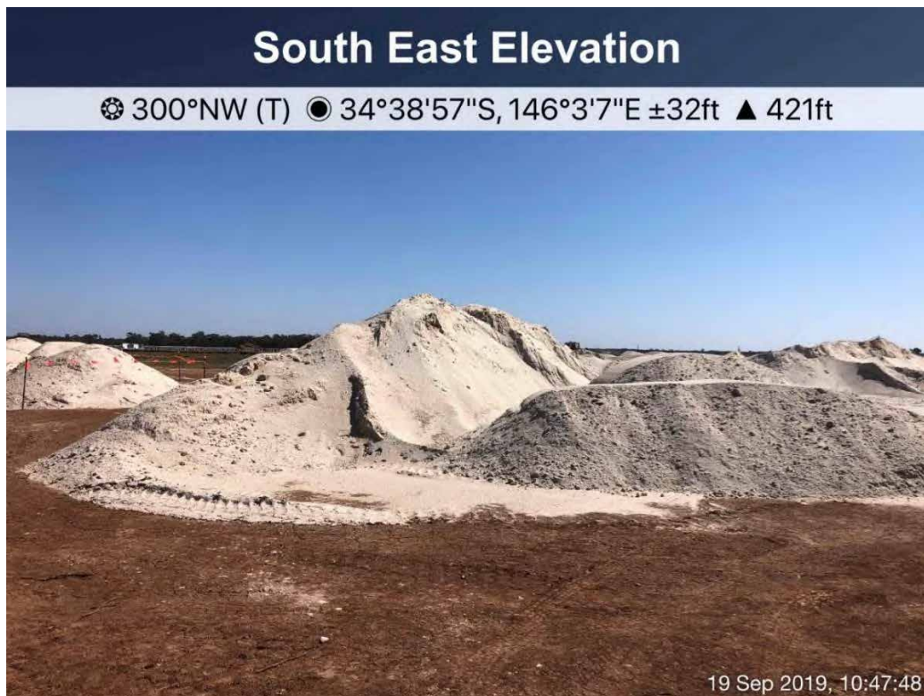
Photograph 58: Sand stockpiles, possibly higher than 2m, not adequately protected with ESC devices
