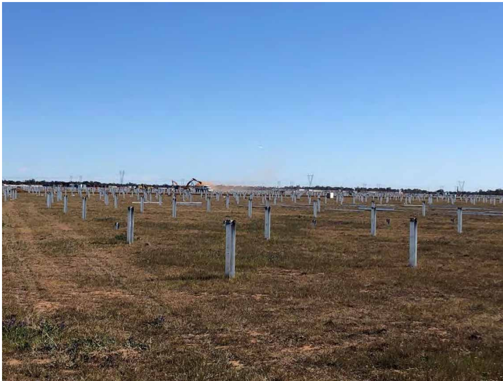
Photograph 8: Example of dust generating activity with no water truck for dust suppression in use, view towards south-west (transmission powerline in background), view of pile installation.
