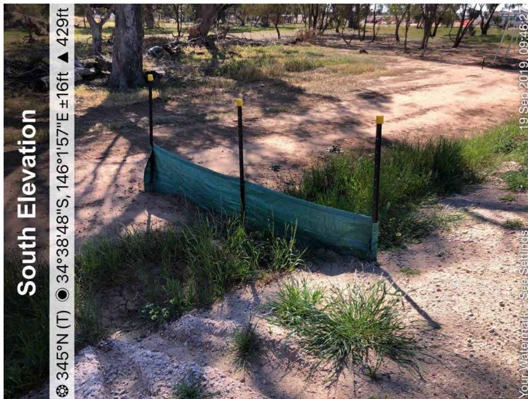
Photograph 50: Northern drain at front entrance, ESC device recommended to remove or replace with rock filter, coir log or hay bale, adequate vegetation to filter runoff
