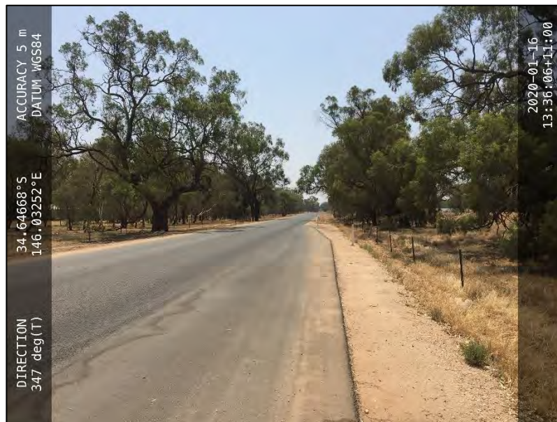
Photograph 10: Facing north along Donald Ross Drive from the DPSF site entry during the day.
