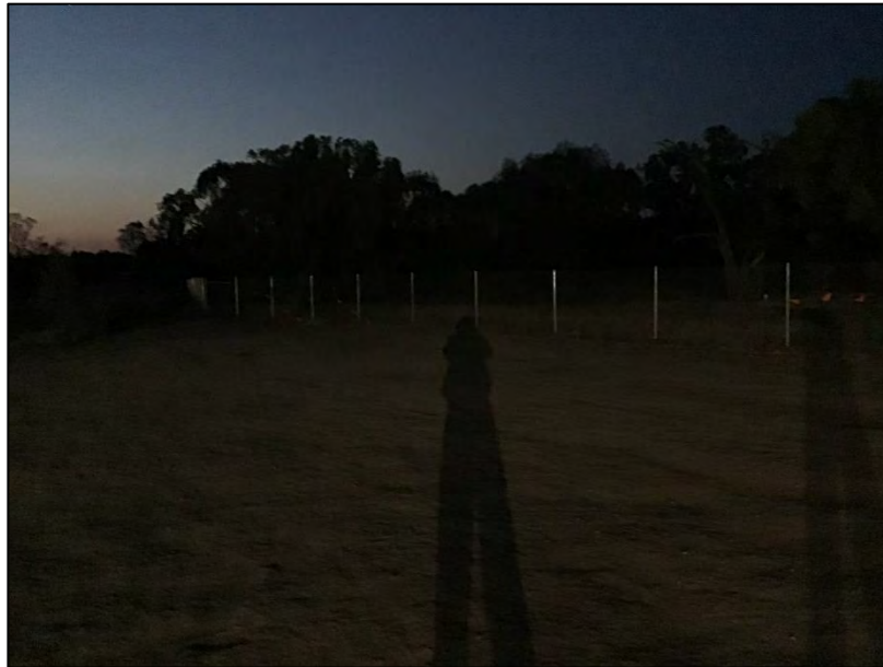
Photograph 4: Interface between the Construction Compound and the Retained Vegetation Parcel north of the DPSF site entry
