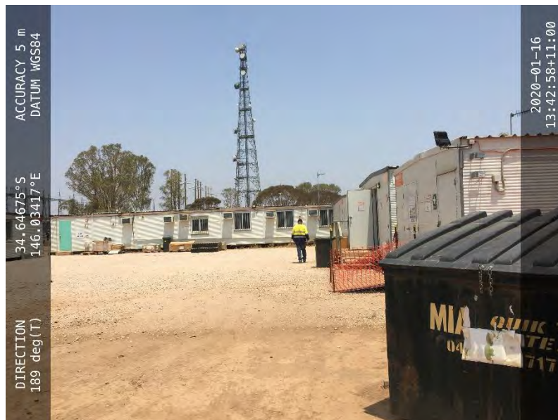
Photograph 9: Security lighting arrangement at the DPSF Construction Compound. Lights face below the horizontal, towards internal areas of the compound (away from external receivers) where not required for access (i.e. lights immediately adjacent to access driveway).
