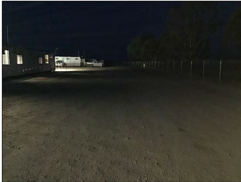
Photograph 6: Interface between the Construction Compound and the northern border of the TransGrid Darling Point Substation at night.
